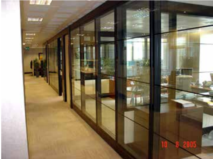
Sound transmission class (STC) of 44 with 2x 6 mm (1/4") laminated glass and 41 with 2x 6 mm (1/4") tempered glass
