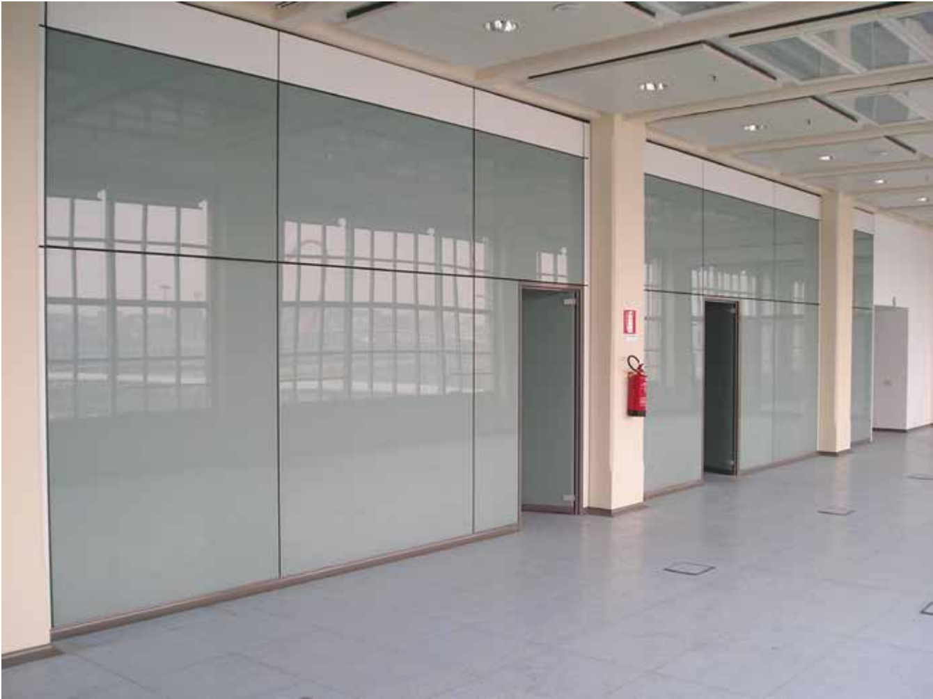
Sound transmission class (STC) of 44 with 2x 6 mm (1/4") laminated glass and 41 with 2x 6 mm (1/4") tempered glass
